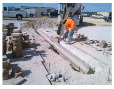
and reinforcing bars. This pour needs to be set firmly before final concrete placement. The required wait time varies with concrete mix design and temperature, but will range from 30 minutes to 48 hours.
