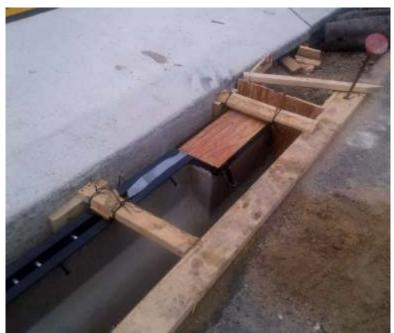
to the outlet (pipe). The trenches should get sequentially smaller the further you move away from the outlet location.
